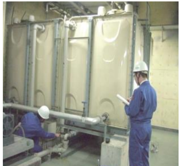
貯水槽の点検
