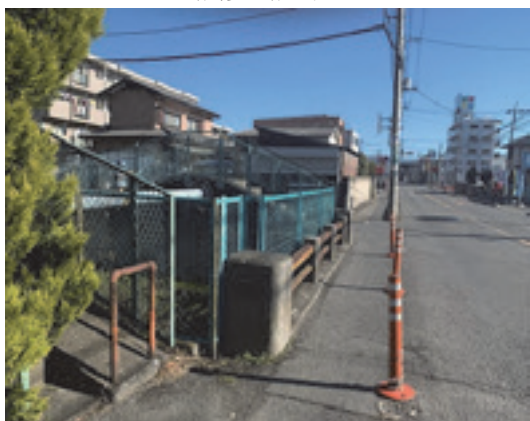
補修・補強前
