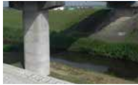
橋梁の耐震補強
