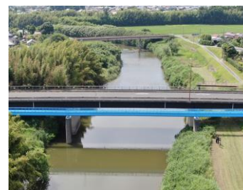
橋梁の耐震補強
